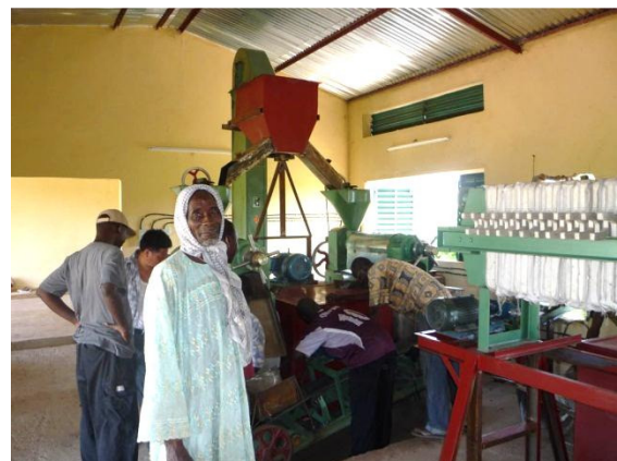
Figure 11: Jatropha pressing hardware installed in Garalo by MFC Nyetaa. The picture shows the village leader Mr Mamadou Kane, the initiator for the electrification of his village [D]
